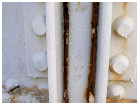
Exterior anchor bolt 17
