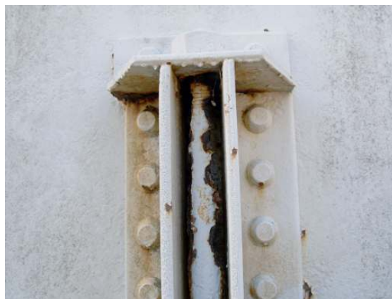
Exterior anchor bolt 1
