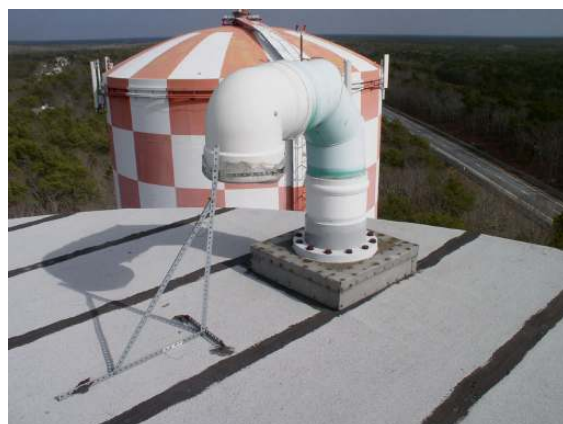
Exterior roof vent 1
