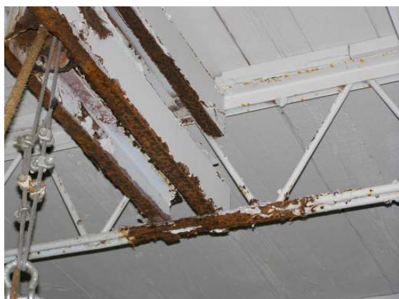
Interior roof framing 3
