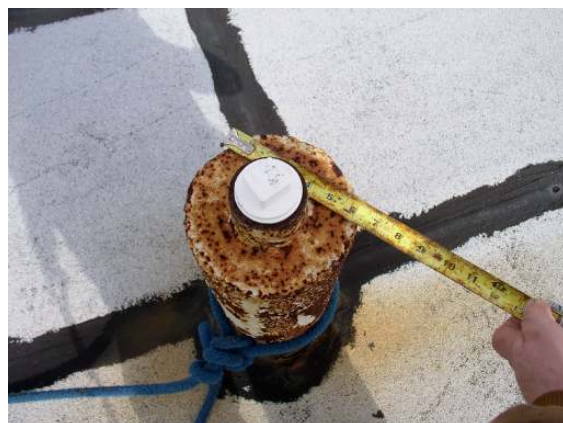
Exterior roof center post 3
