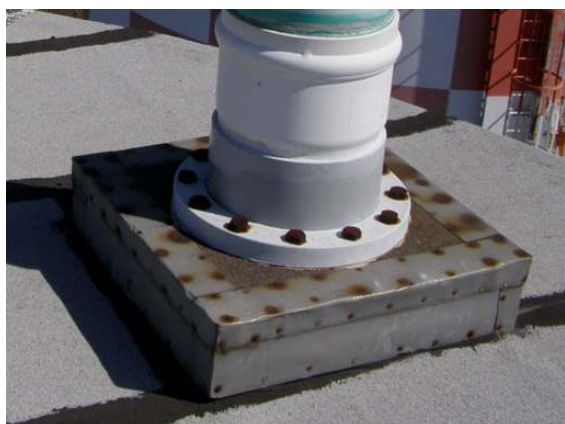
Exterior roof vent 6
