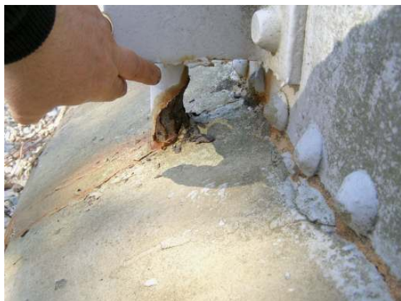
Exterior anchor bolt 18
