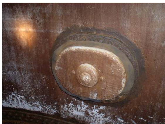
Interior shell manhole 1
