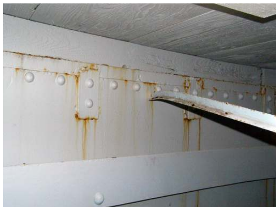
Interior roof to shell junction 1
