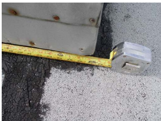
Exterior roof hatch 6
