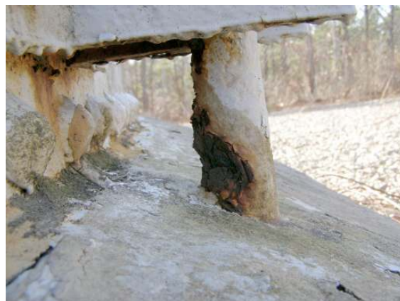
Exterior anchor bolt 13
