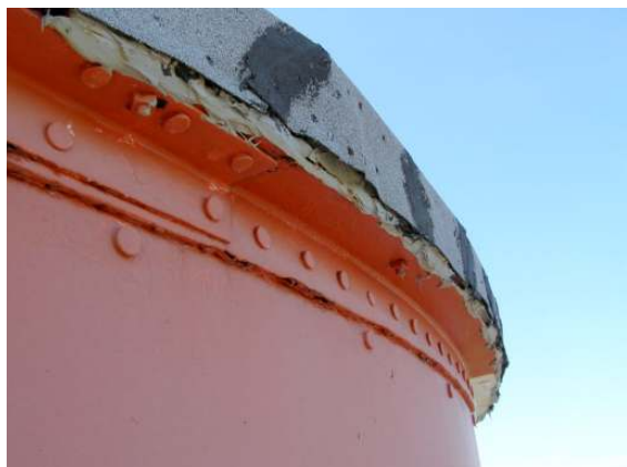
Exterior roof to shell angle 3
