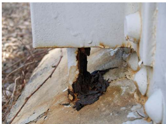
Exterior anchor bolt 10
