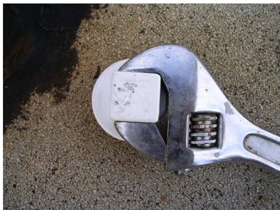
Exterior roof center post 10
