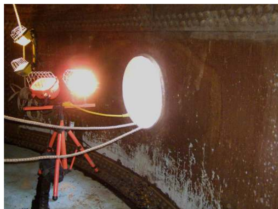
Interior shell manhole 3
