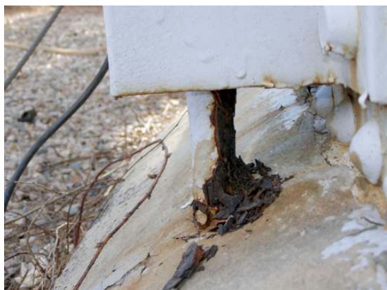
Exterior anchor bolt 16
