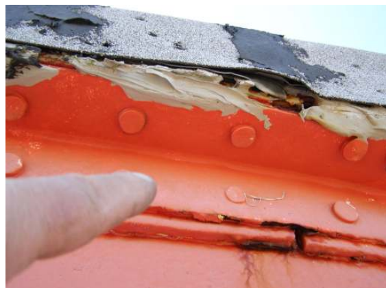
Exterior roof to shell angle 4
