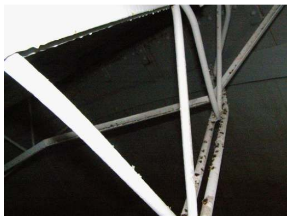
Interior roof framing 10
