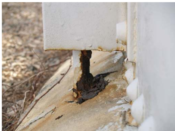
Exterior anchor bolt 12
