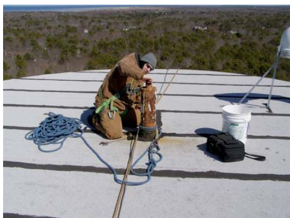
Exterior roof center post 12
