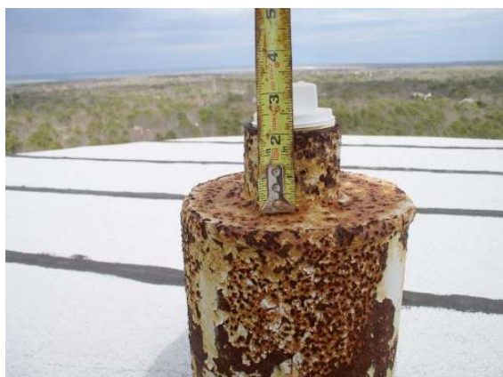
Exterior roof center post 6
