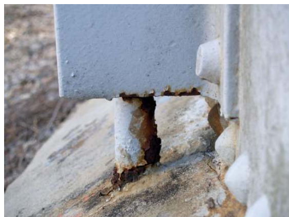
Exterior anchor bolt 11
