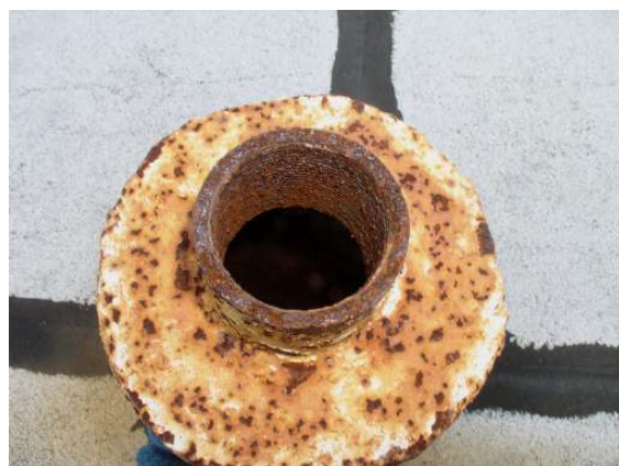
Exterior roof center post 7
