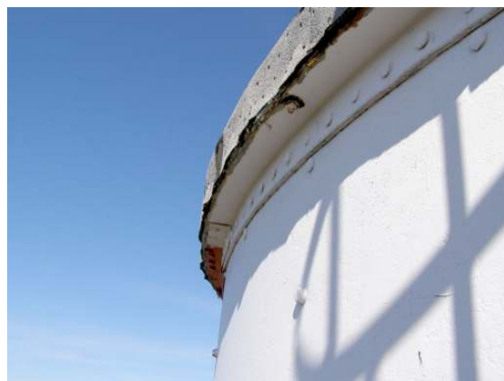
Exterior roof to shell angle 2
