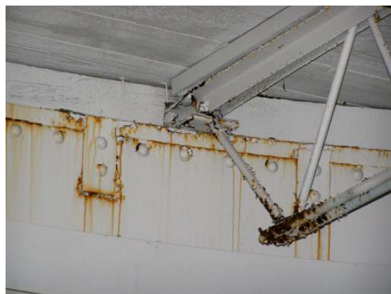
Interior roof framing 6
