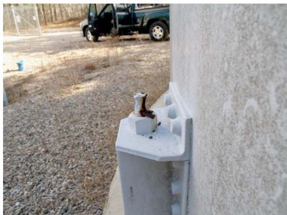
Exterior anchor bolt 6
