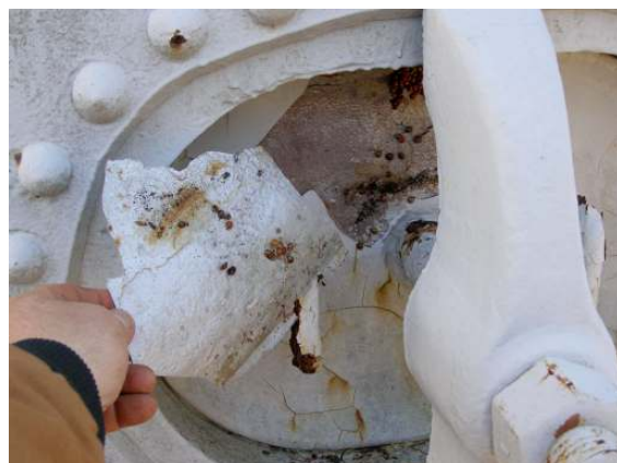
Exterior shell manhole 3
