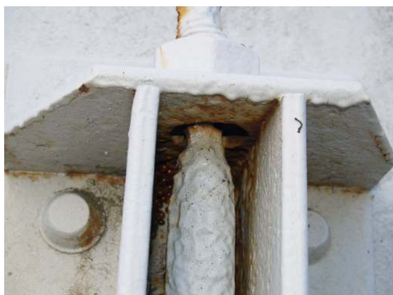
Exterior anchor bolt 8
