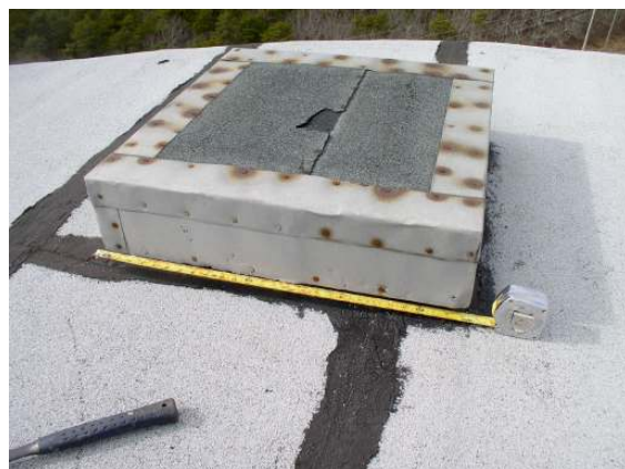
Exterior roof hatch 3
