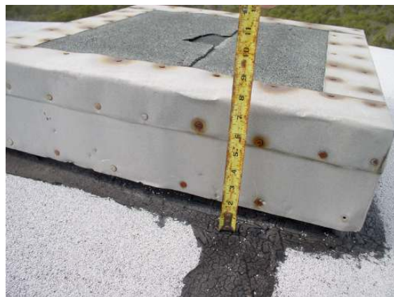
Exterior roof hatch 5
