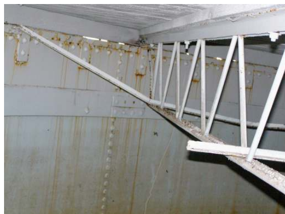
Interior roof framing 12
