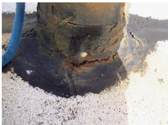
Exterior roof center post 8
