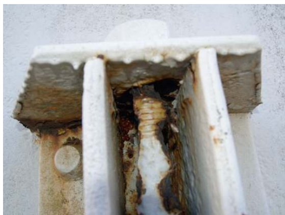
Exterior anchor bolt 4
