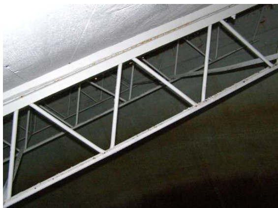
Interior roof framing 11
