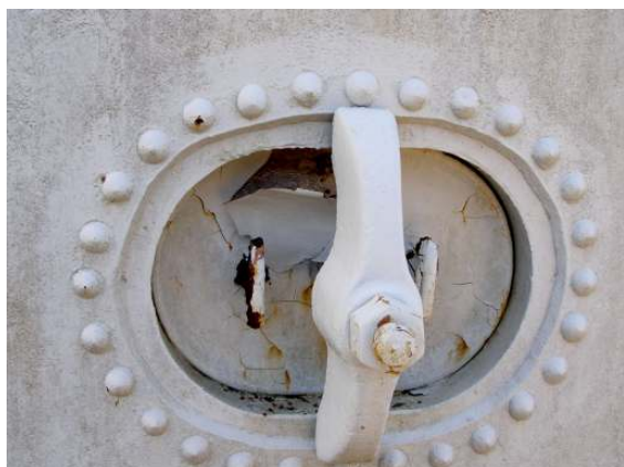
Exterior shell manhole 2
