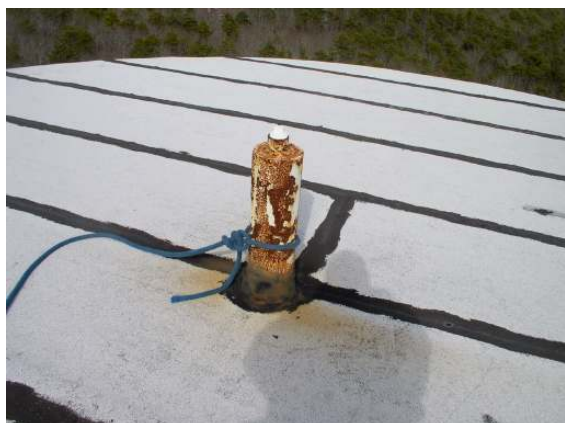
Exterior roof center post 2
