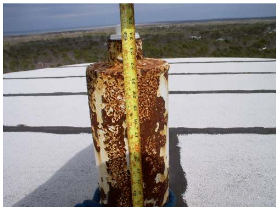
Exterior roof center post 4
