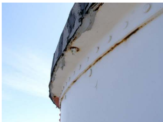
Exterior roof to shell angle 5
