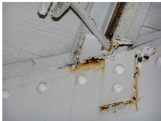
Interior roof framing 8
