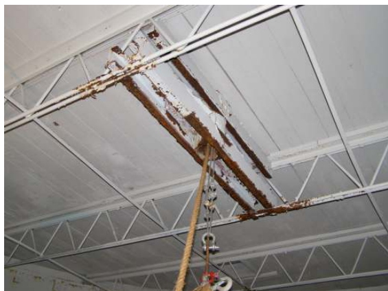
Interior roof framing 1
