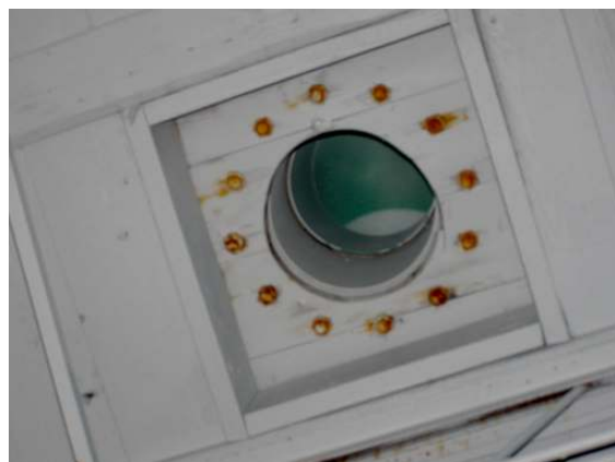
Exterior roof vent 3
