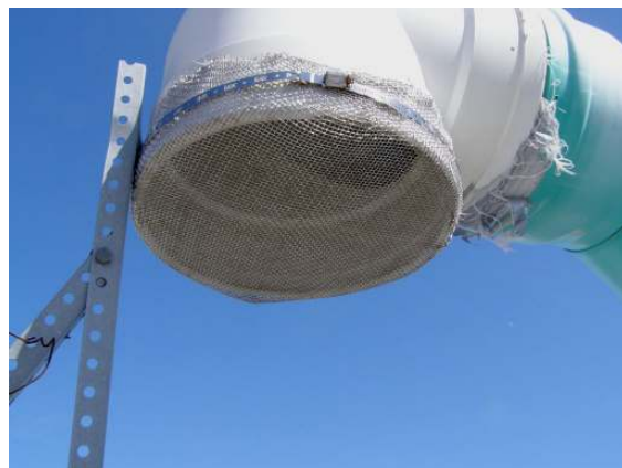
Exterior roof vent 5
