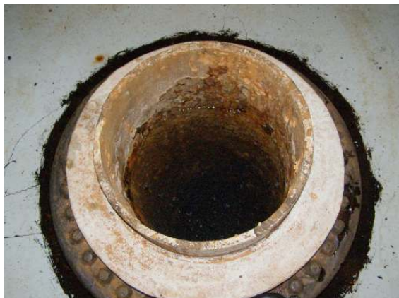
Interior silt stop 2
