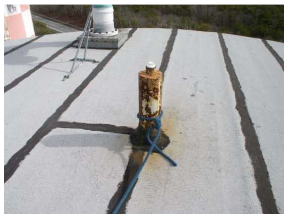
Exterior roof center post 1
