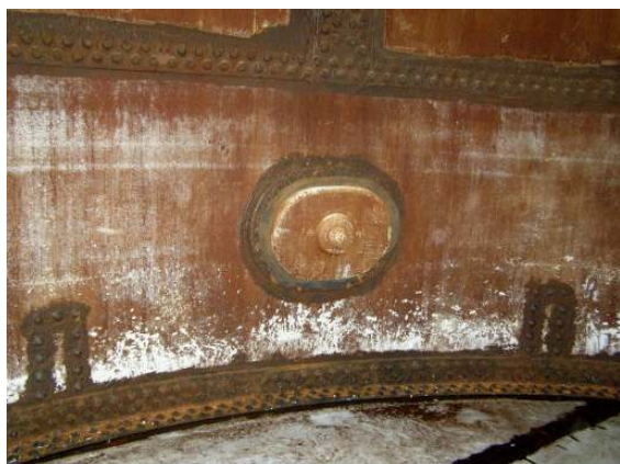
Interior shell manhole 2
