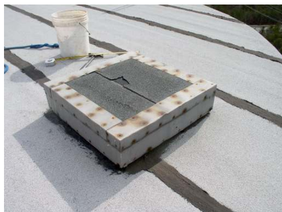
Exterior roof hatch 1
