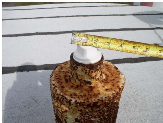
Exterior roof center post 5
