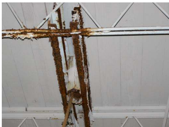
Interior roof framing 5
