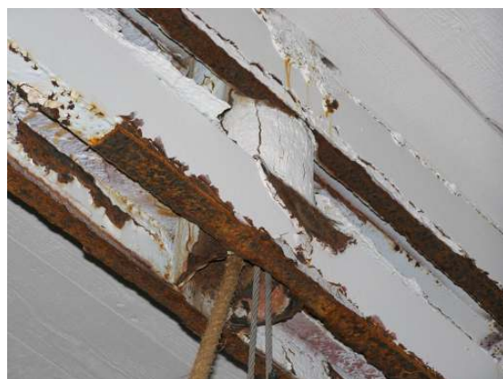
Interior roof framing 4
