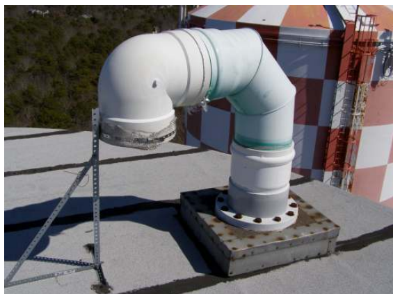
Exterior roof vent 4
