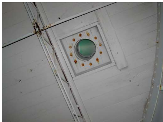
Exterior roof vent 2
