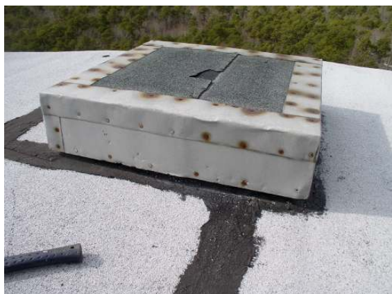
Exterior roof hatch 2
