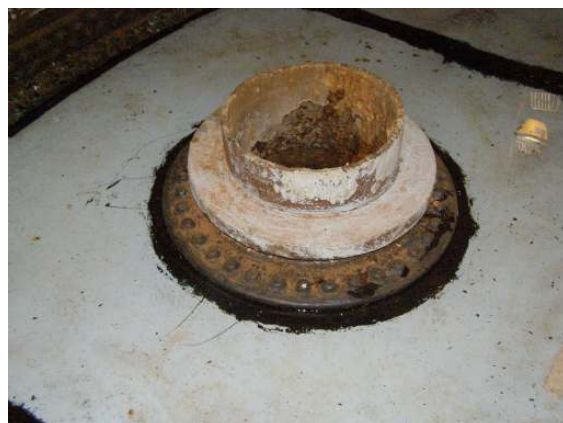
Interior silt stop 1
