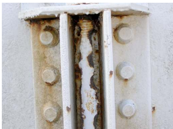
Exterior anchor bolt 14
