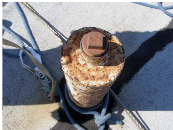
Exterior roof center post 11
