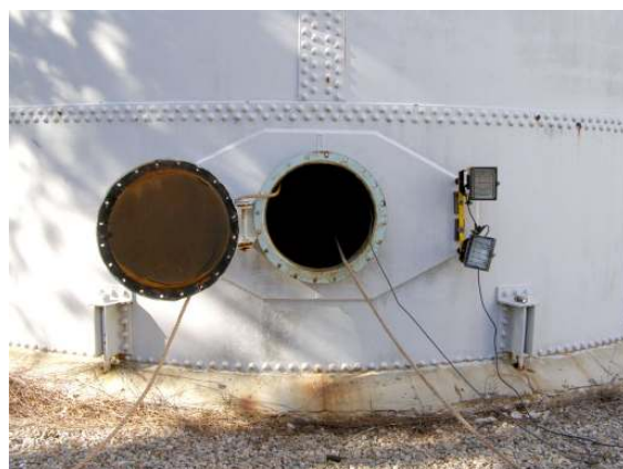
Exterior shell manhole 1
