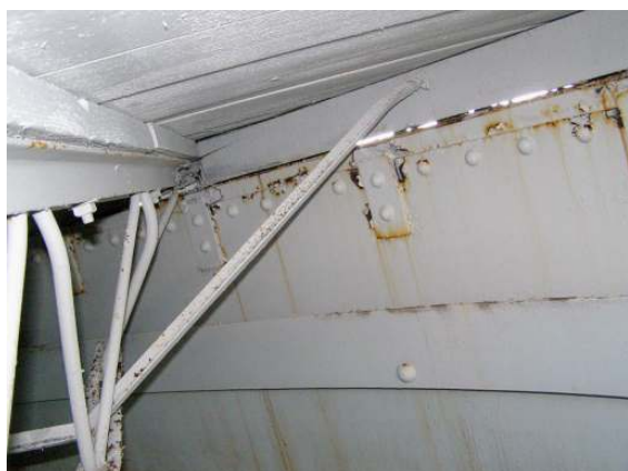
Interior roof framing 9
