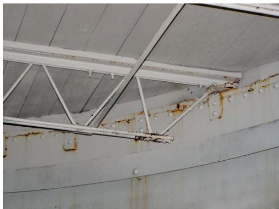
Interior roof framing 7
