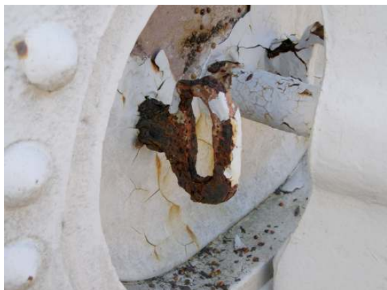
Exterior shell manhole 4
