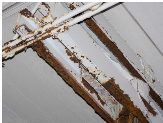
Interior roof framing 2
