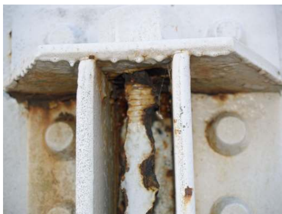
Exterior anchor bolt 2
