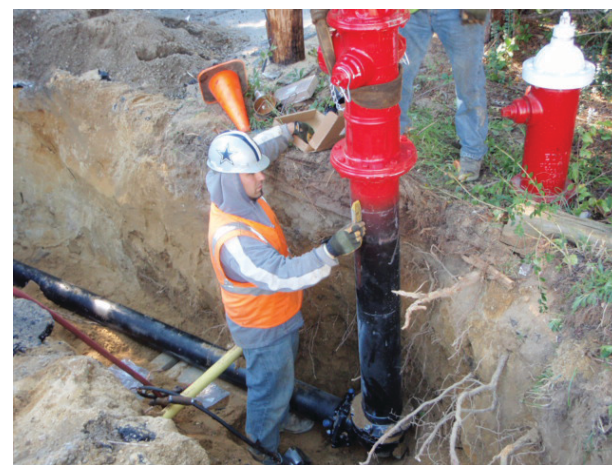
Replacement of a deficient fire hydrant
