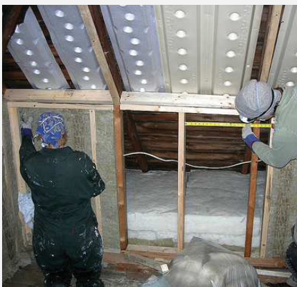
a) Building Retrofits
