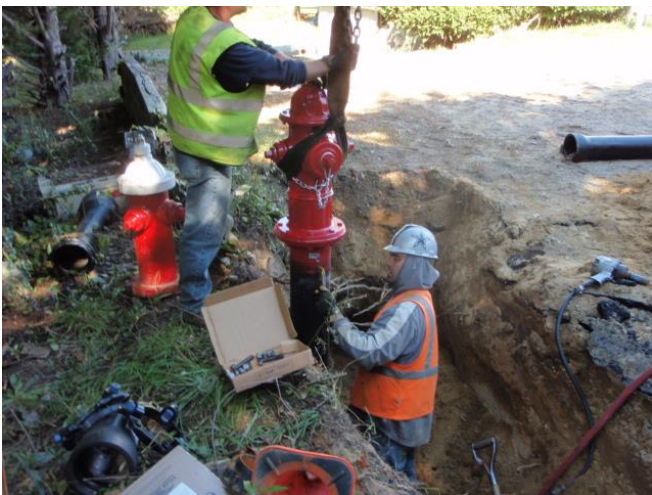
Public Fire Hydrant Installation
