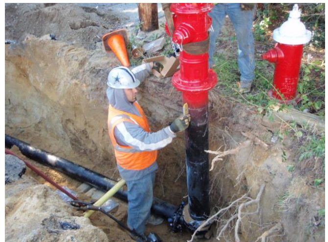
Public Fire Hydrant Installation
