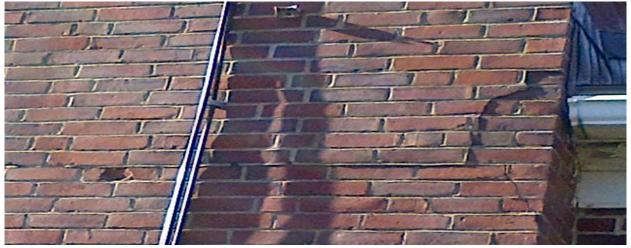
**BCHMCPS Exterior Photos: (Cracked mortar, bulging wall)**
