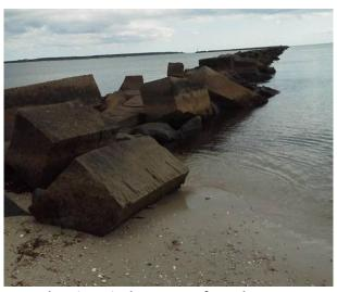
**Showing Displacement of Breakwater Stones**
