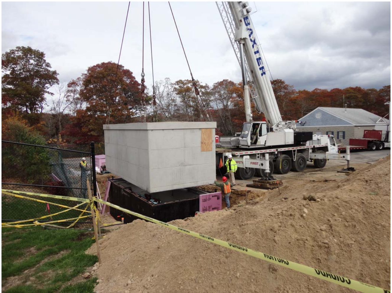
Straightway Pump Station Installation
