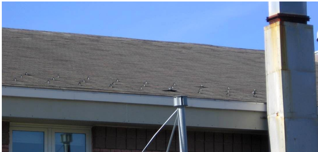
Sloped roof shingle damage (missing tabs) throughout entire roof area.
