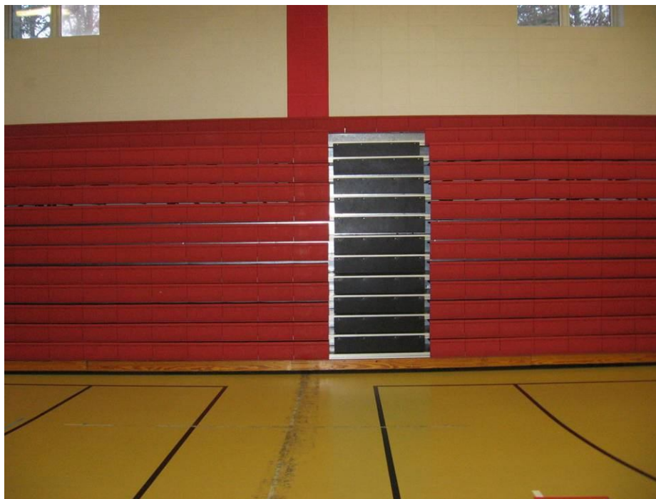
Bleacher in closed position. Note floor damage due to faulty mechanism.
