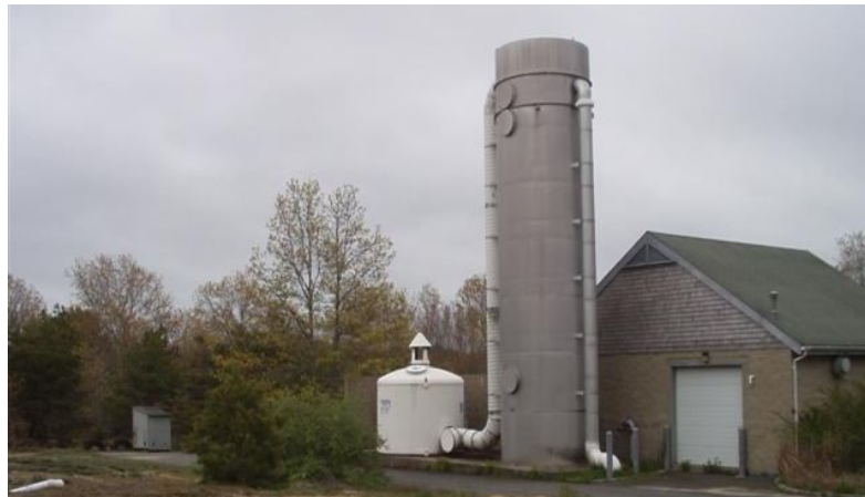
Maher Treatment Plant
