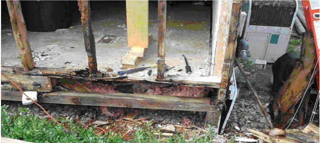
Rot in corner of existing building
