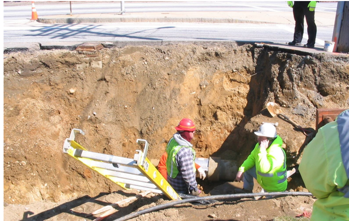
Installing new water pipes
