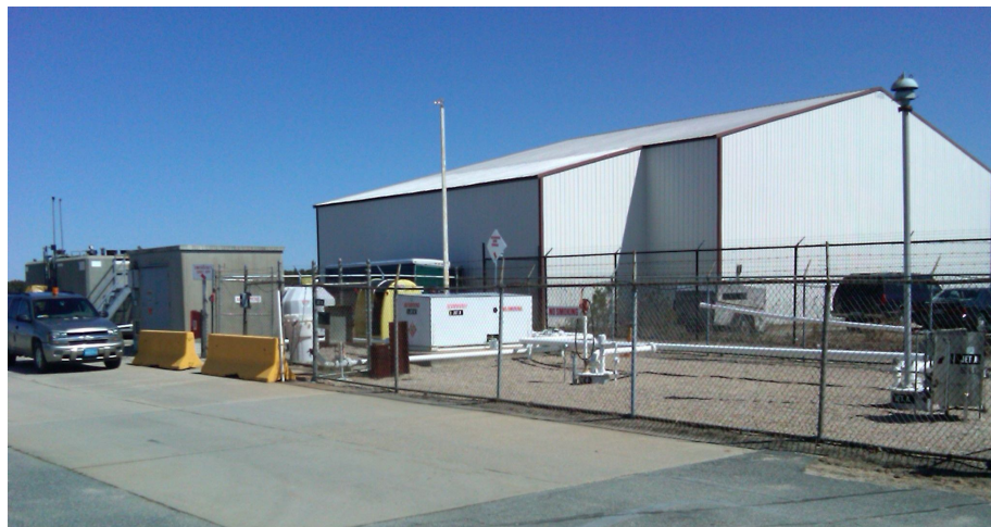
Existing Fuel Farm
