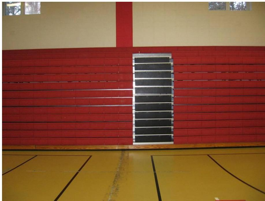
**Bleacher in closed position. Note floor damage due to faulty mechanism.**
