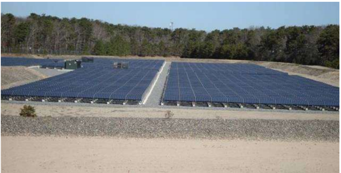
Solar Array at the Water Pollution Control Facility
