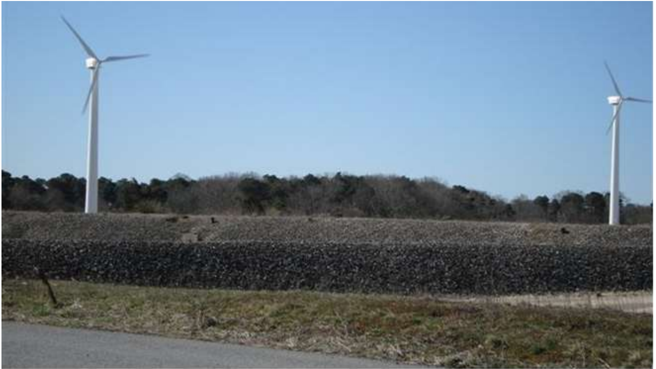
Wind Turbines at the Water Pollution Control Facility
