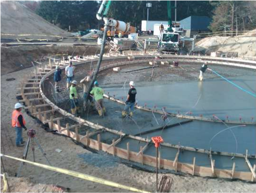
Construction of new Maher Water Tank
