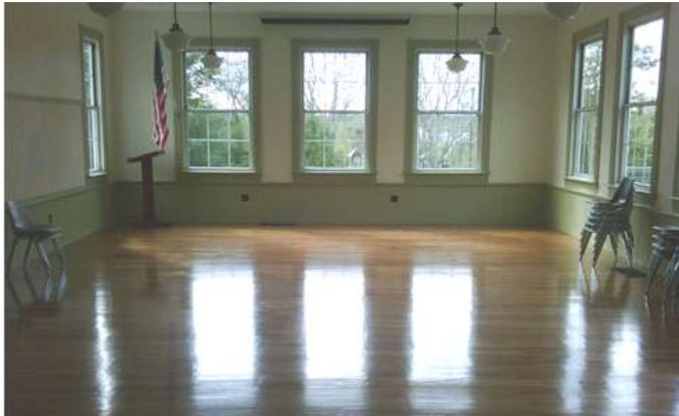
West Barnstable Community Building Floor Refinishing
