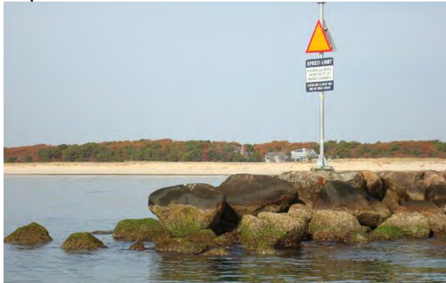
West Bay Breakwater
