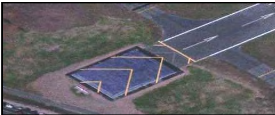
Engineered Material Arresting System (EMAS) bed
