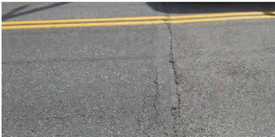
Bumps River Bridge – Surface Cracking
