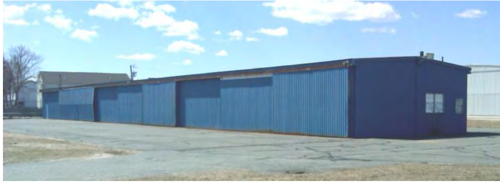
Existing T Hangar
