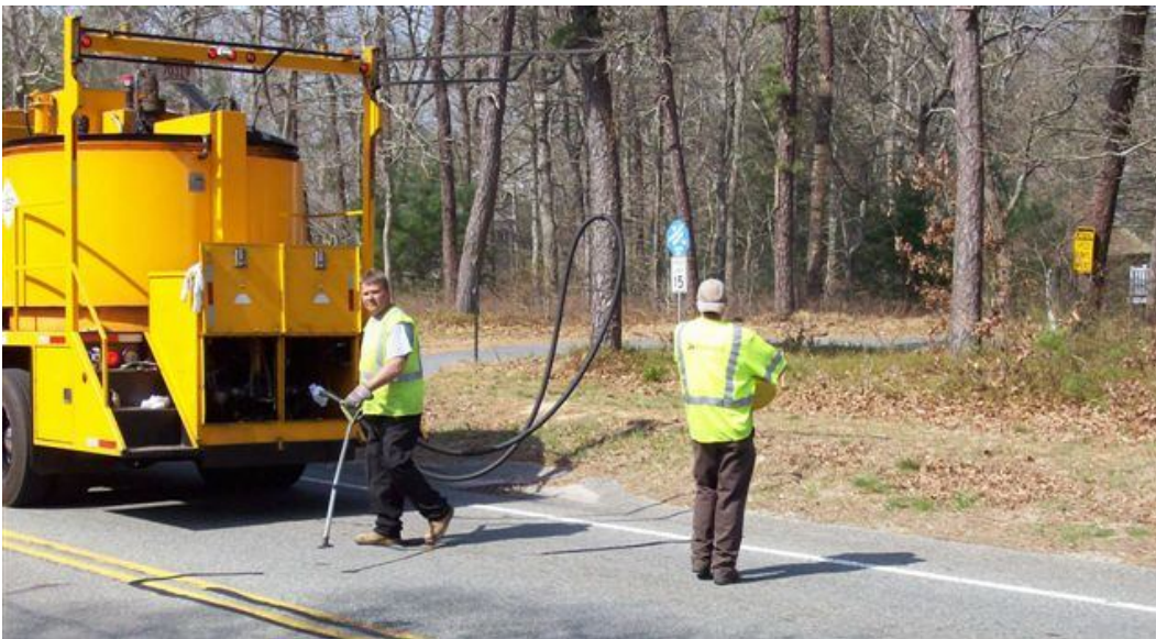
Crack Sealing Phinney's Lane
