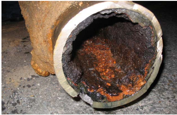
Cast Iron Water Pipe Corner Main & Pleasant Streets Hyannis
