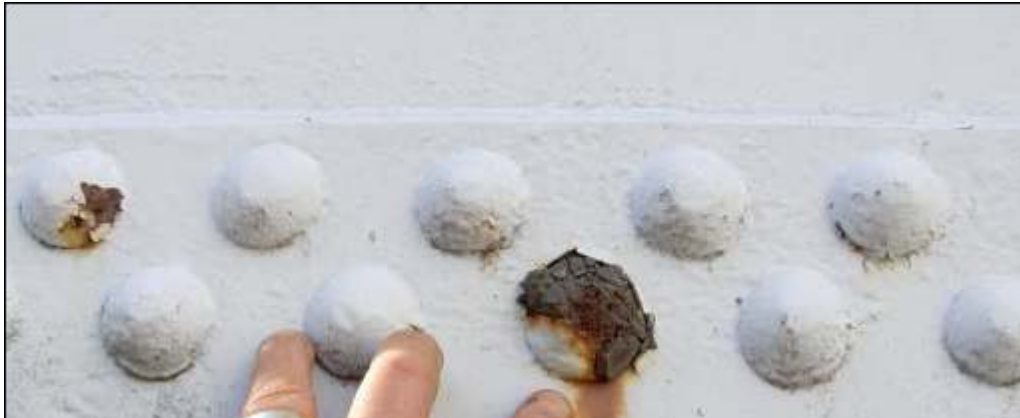
Deteriorated Exterior Rivets Mary Dunn Water Tank
