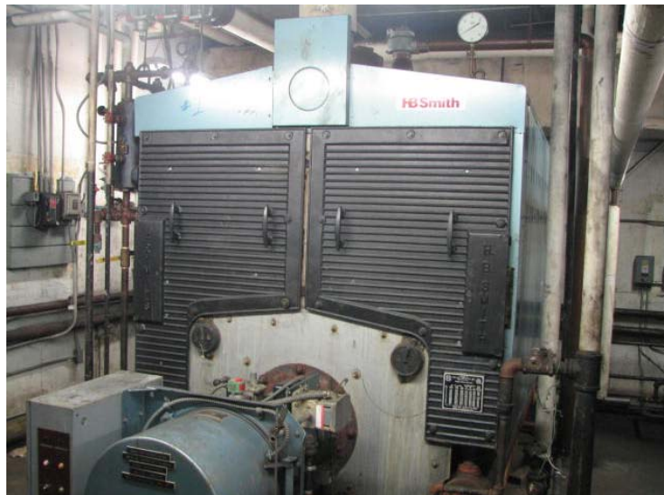
Centerville School Boiler
