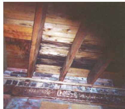
Deterioration Below the SAB Roof
